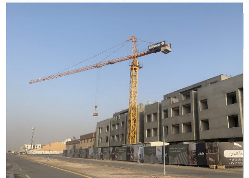
03 Turnkey Construction Riyadh, KSA 2022-2023 View Project Corporate
