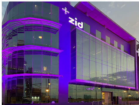
02 ZID Full Fit Out Replacement Riyadh, KSA 2022-2023 View Project Corporate
